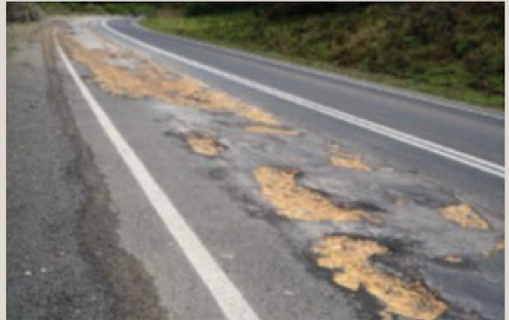
Figure 6: Failure of the road surface on Portland Nelson Road due to increasing truck volumes
