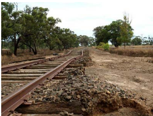
Flood Damage to Mallee Rail Network 2011 Photo: Cr Cliff Unger, Mayor Hindmarsh Shire
