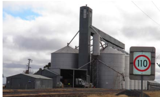
Grain trucks unloading at Wycheproof Bulk Terminal
