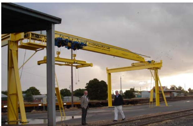
Peaco Rail Loading Facility at Donald
