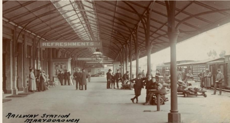
Maryborough Station in its heyday, c1890s, "a railway station with a town attached" – attributed to Mark Twain, 1895. This station has recently undergone a major refurbishment to provide a new tourist and community hub. Our InterCity blueprint would recreate it as a transport hub.
