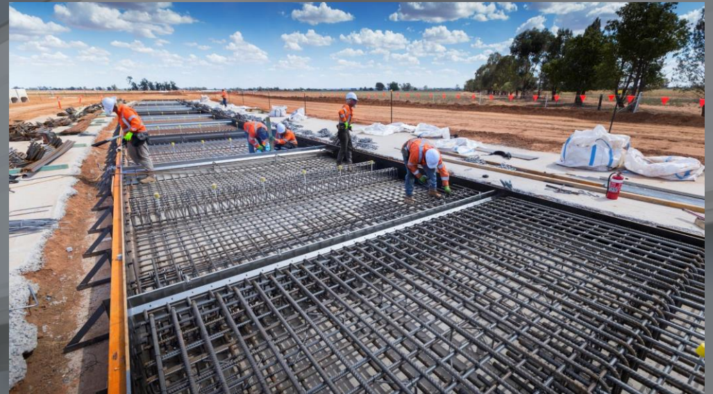
Base for new culverts
