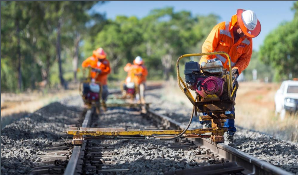
Unclipping the old rail
